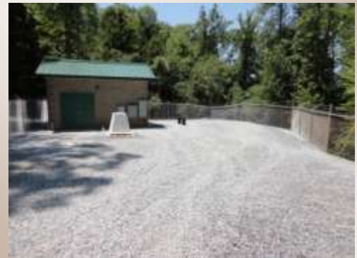
Pump & Treatment Facility
