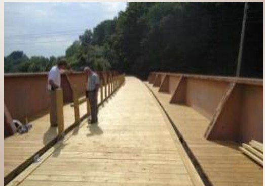
Milligan Hwy. Bridge During
